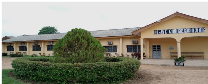
Plate 4: Approach View of Department of Architecture building (LAUTECH)
