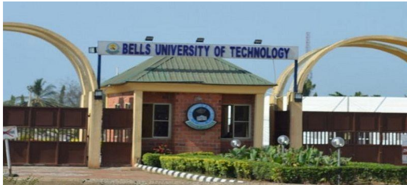
Plate 6: Entrance gate of Bells University of Technology
