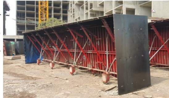
Figure 2:- Tunnel Form and its components
