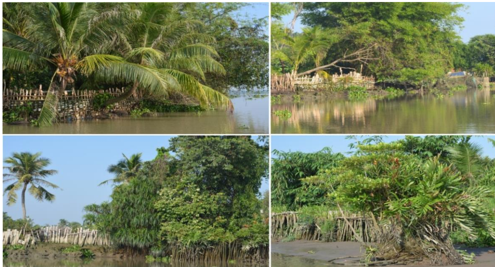
Figure 4. The anti-erosion works along Rach Tra
