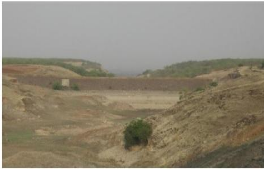
Photo-2- Progress of work on Site for-Percolation tank
