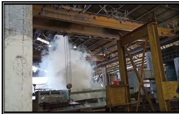
Figure 3: Toxic fumes emerging from the tank and going towards the VFD panel.
