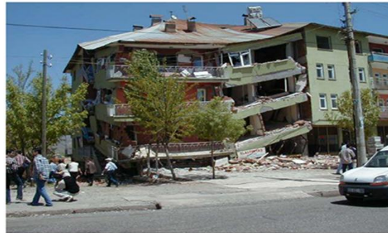
Fig 1: Adjacent buildings fail during the Bingöl earthquake (source: Ahmet Topçu).
