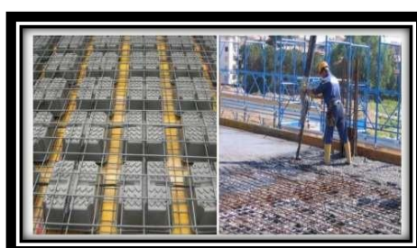
Fig 3. Installation of U-Boot Beton
