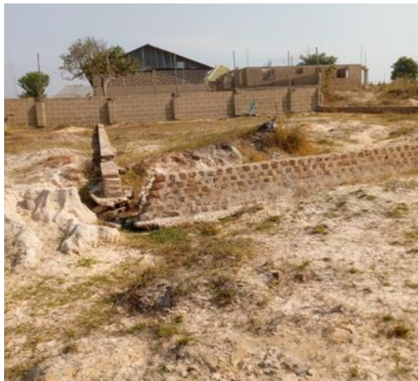
Figure 5: Evidence of sand excavation on building at Tse Poor.
