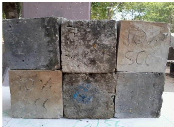
Figure 3.2: Chloride attacked concrete cubes
