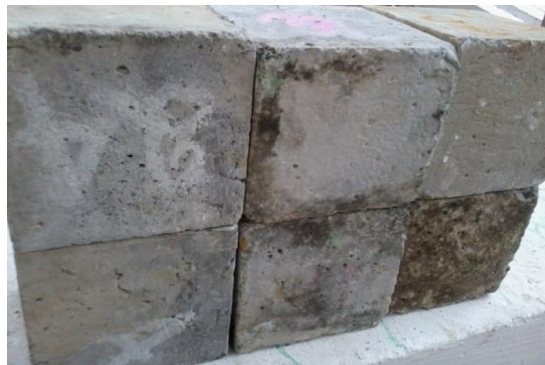
Figure 3.1: Acid attacked concrete cubes
