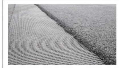
Fig 4: Fiberglass geogrid
