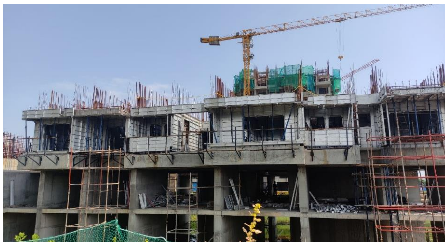
Figure 1.1: Building Construction with Mivan Method
