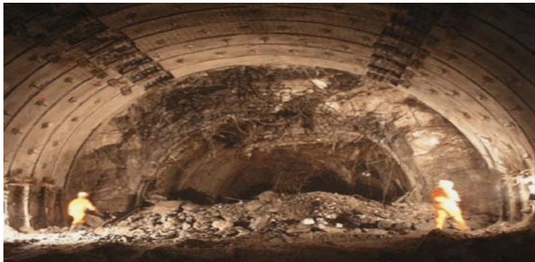
Fig-2: Conventional tunneling of GBT
