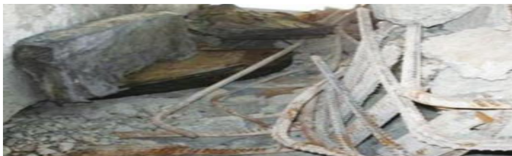
Figure 7: Damaged Bearing
