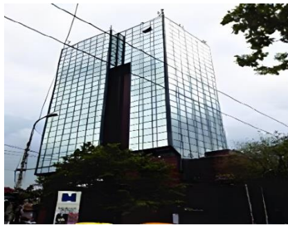
Fig 1. Office structure under examination
