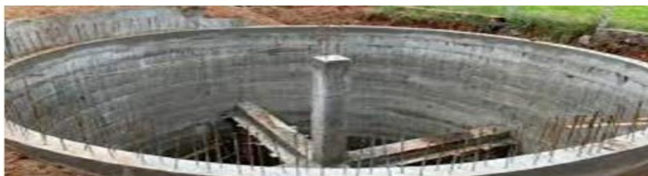
Fig. 1.1 Underground Circular Water Tanks
