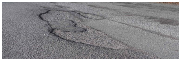
Figure i) Delamination
