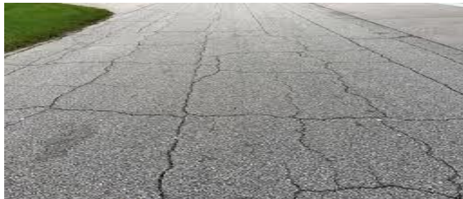
Figure c) block cracking
