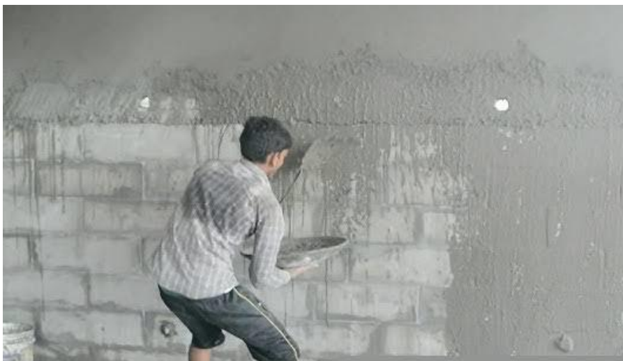
AAC Block wall plastering
