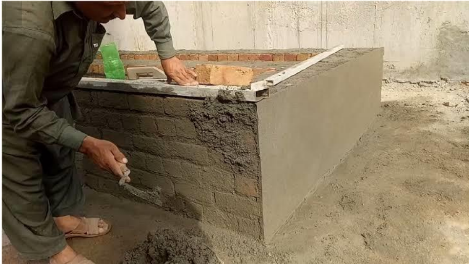
Brick wall plastering
