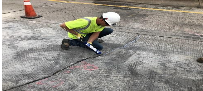
Fig.(c) Routing and sealing pavement cracks.
