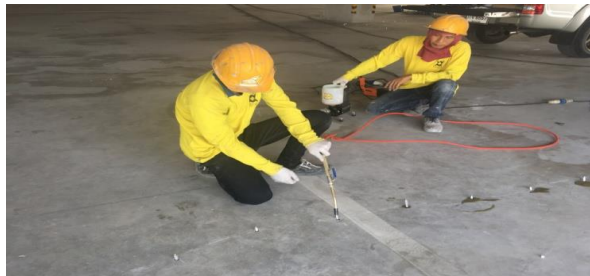
Fig.(a) Concrete Structure Crack repair by epoxy injection.
