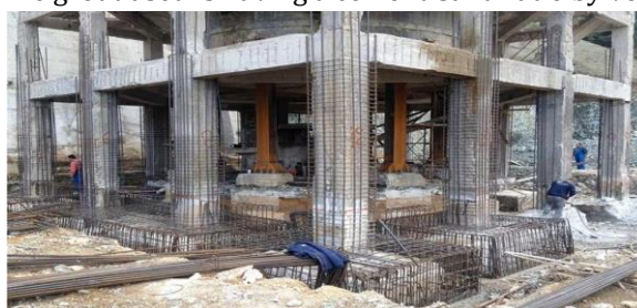
Fig.(b) Jacketing of reinforced concrete (RC) columns.
