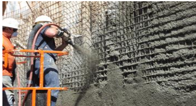
Fig.(d) Shotcrete work.
