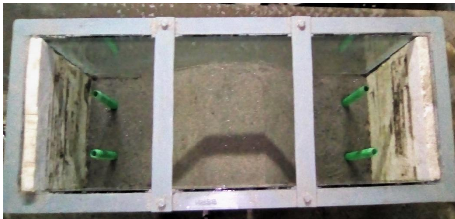
Fig.-4: Installation of perforated pipes in the tank for grouting
